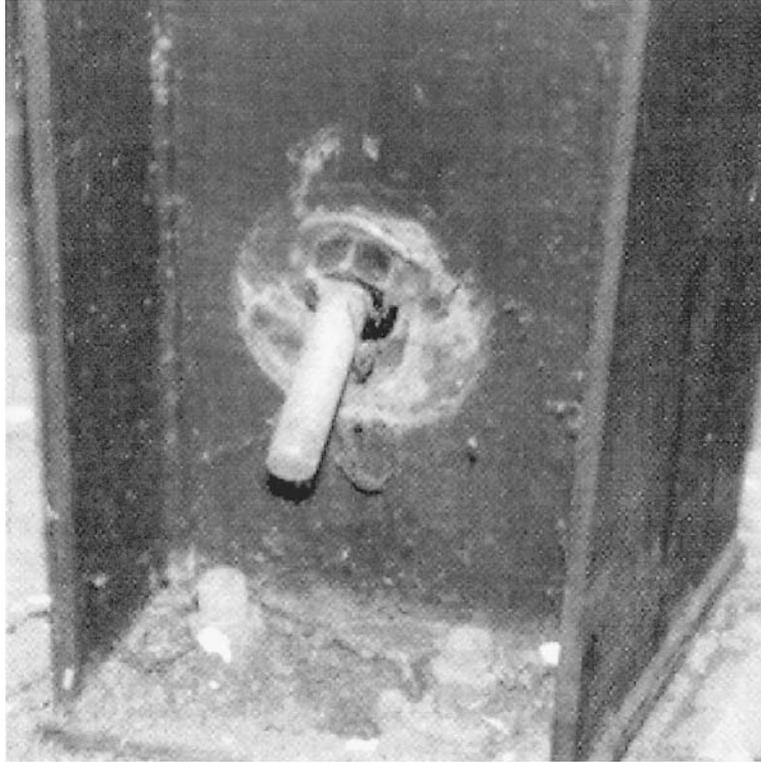
**FIGURE 3.15** This is where a hillside washer was before the Northridge earthquake. (*J. R. Miller & Associates.*)
